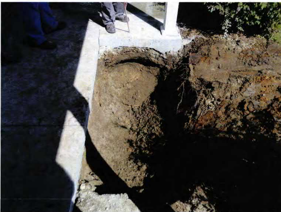
Picture 2: UST 428Elderberry excavation.
